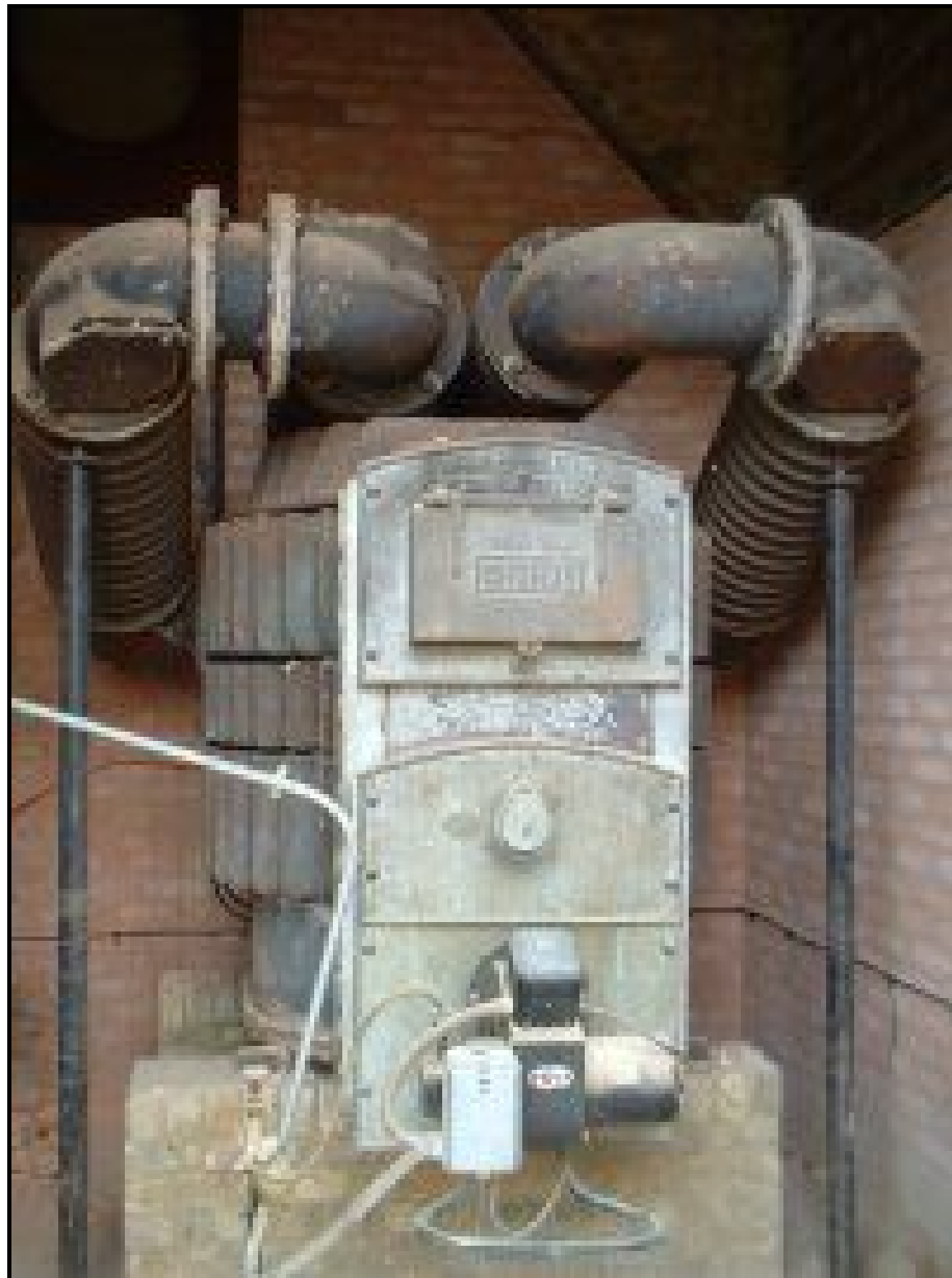
Grundy stove before removal at St Barnabas in Epsom
